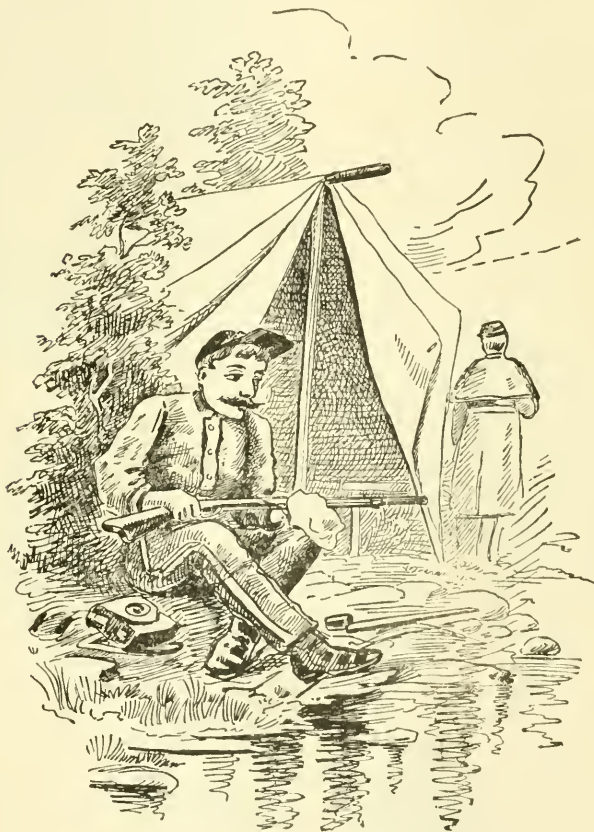
GETTING READY FOR INSPECTION.
