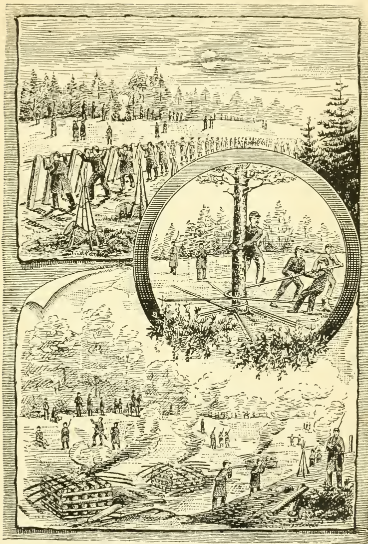
TEARING UP THE WELDON RAILROAD.
